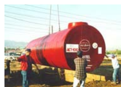
Underground storage tank
